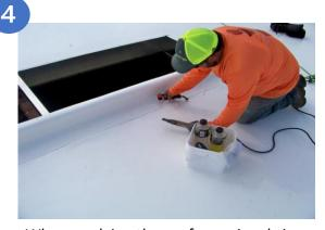
When applying the roof covering, bring it over the top portion of the flashing & secure it down.
