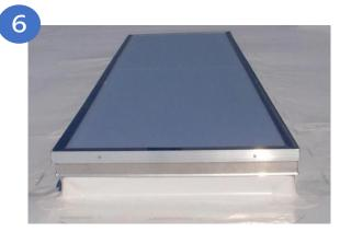
Install the skylight over the finished insulated curb & secure.
