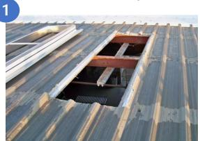
Remove old fiberglass lighting panel & clear away any debris & screws that surround the edges of the opening.
