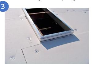
Apply the flute fill & fasten down the insulated board on the roof & apply insulation to the sides of the flashing.
