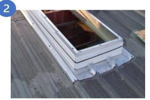
Place the Retro Fit Roof Flashing over the opening. Secure with screws all the way around the flashing.
