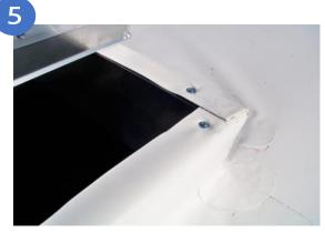
Cover the top of the flashing, secure & trim away any excess material.
